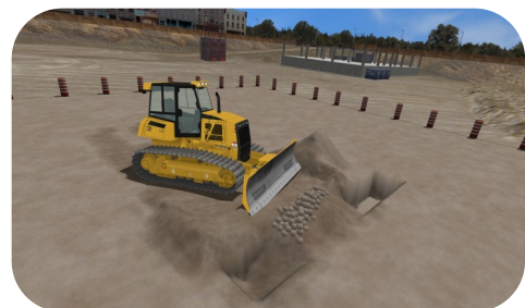
Using the blade to backfill a trench
